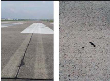
**Above Left:** Figure 2 – marks of hydroplaning on the runway. **Above Right:** Figure 3 – Rubber dumped from tyre.
