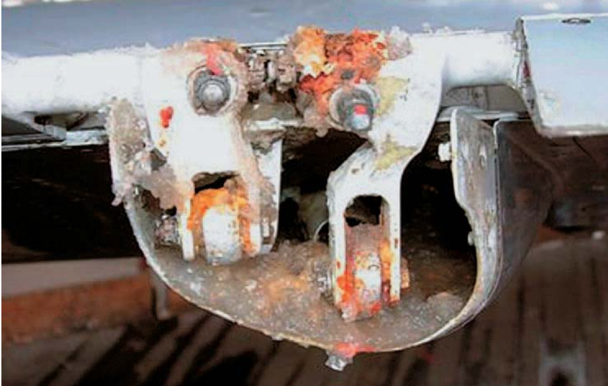
Figure 1: Elevator control maintenance and ground crews should establish an inspection and cleaning schedule for deicing/anti-icing fluid residue to help ensure that no flight control restrictions will occur.
